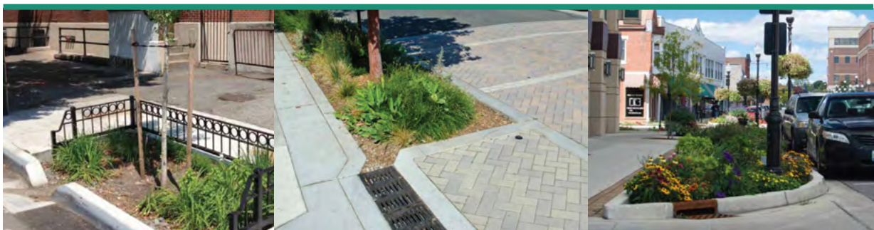
STORMWATER TREES | In this example, a single stormwater tree manages a portion of runoff from the street right-of-way. A single curb cut conveys water from the street into the bed of the planter.
