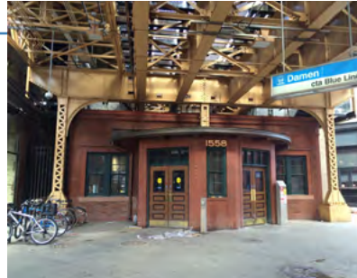
CTA 'Damen' Blue Line Station
