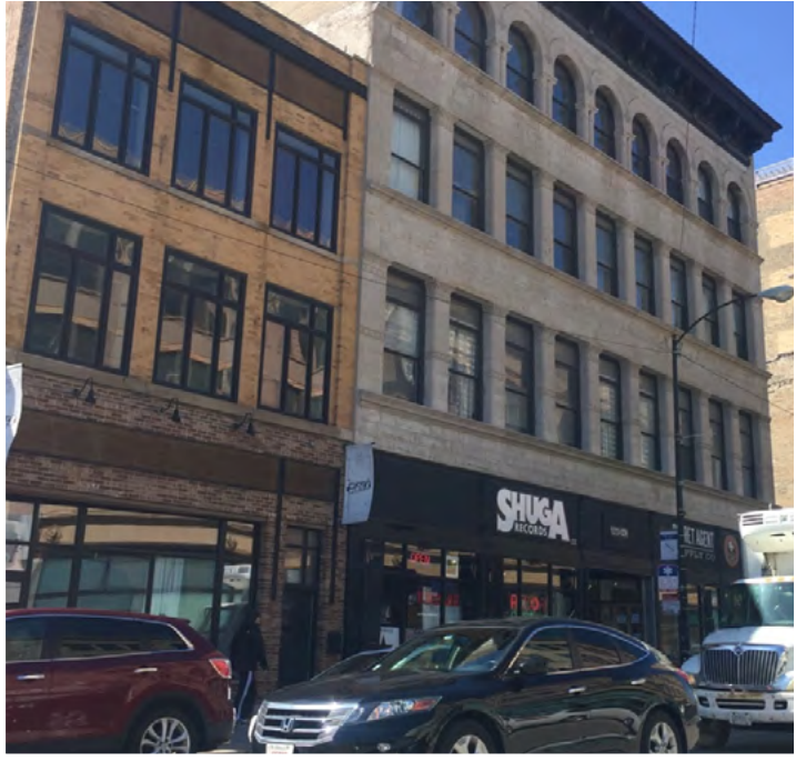
Sensitive renovations of buildings along Milwaukee Avenue have returned residential uses on upper stories and commercial frontages.
