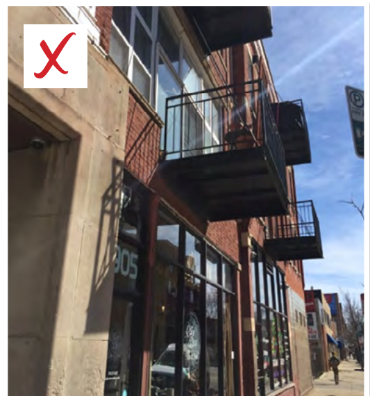
Balconies on rehabbed or new buildings should not intrude over the public right-of-way where passers-by walk on sidewalks.
