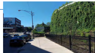
Access to the 606 off of Ashland Avenue
