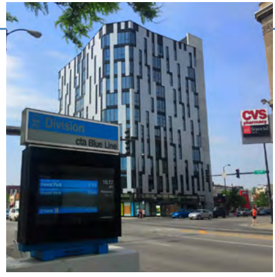
Fifteen-story TOD located at the intersection of Division Street and Ashland Avenue
