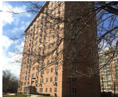
Wicker Park Apartments (Senior Housing) located at 1414 N. Damen
